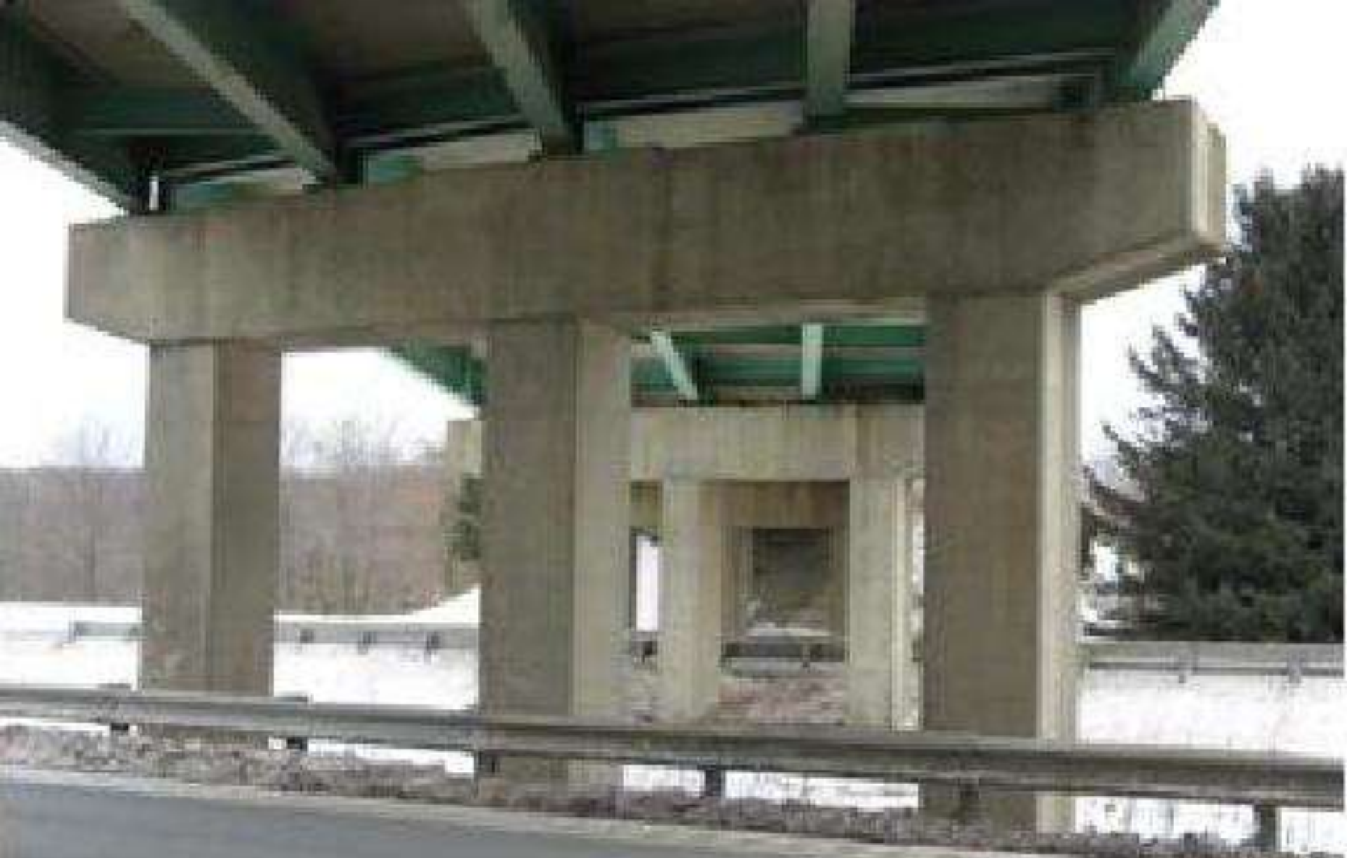
Concrete Column and Cap
